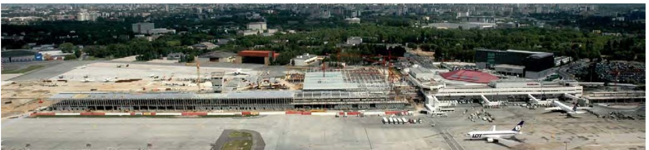
New terminal in Warsaw (Poland)
