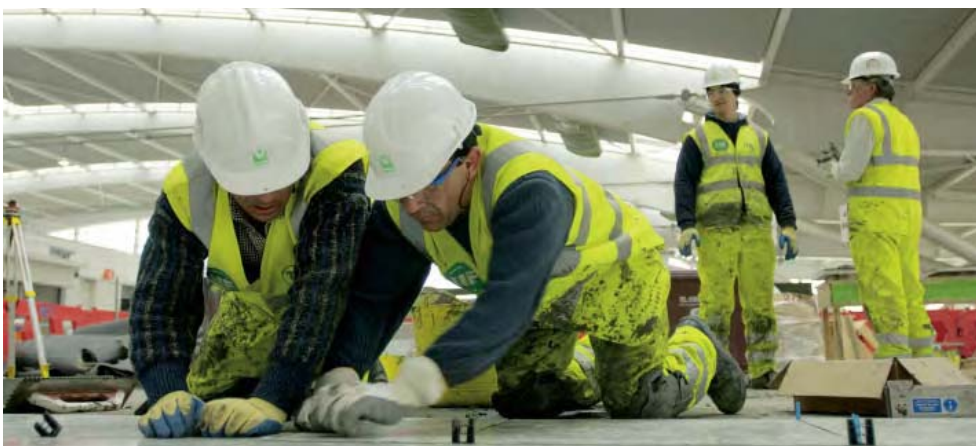
Workers at Heathrow Airport Terminal 5 (London, UK)
