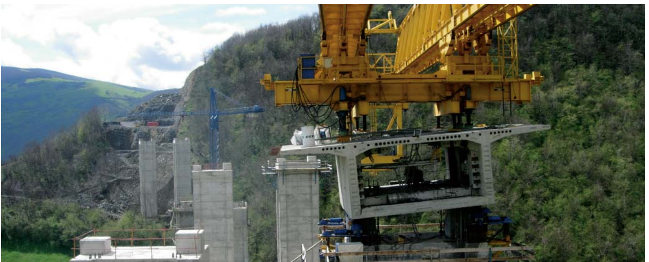
Cantabria-La Meseta trunk road (Spain)
