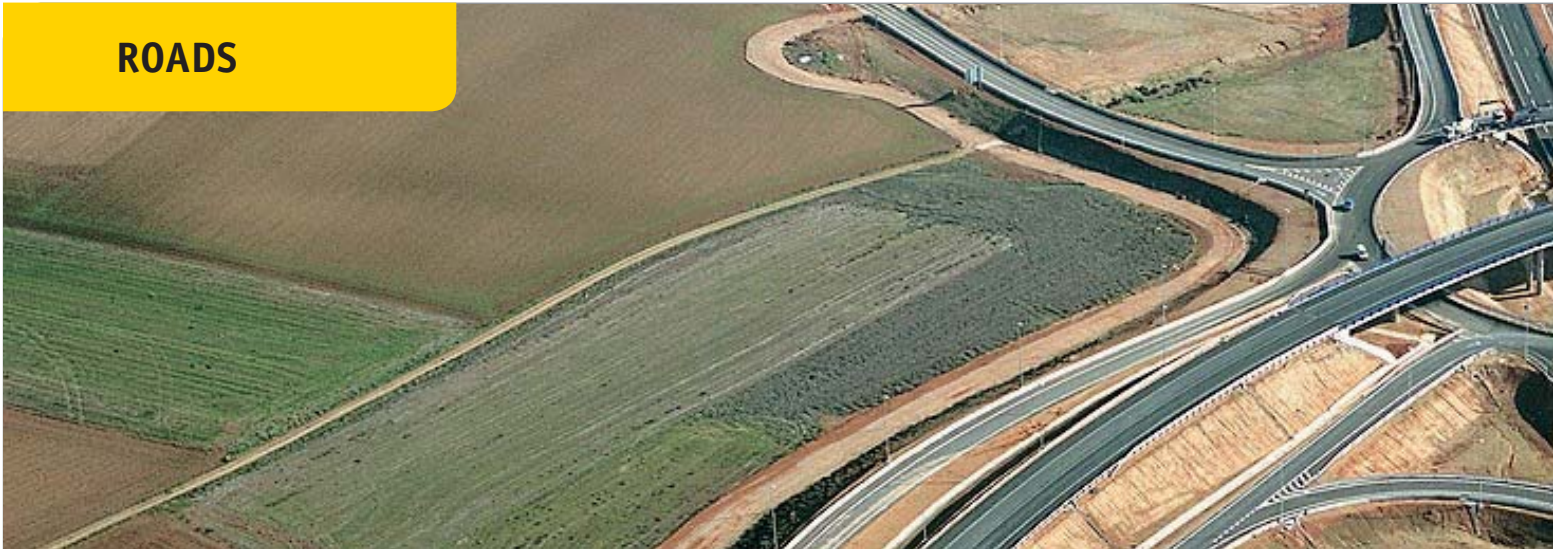
Ocaña - La Roda Toll Road (Spain)
