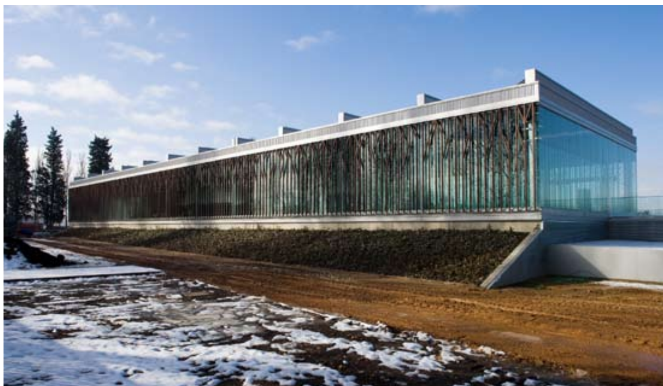
Environmental Resource Center, built by Ferrovial Agromán (Valladolid, Spain)
