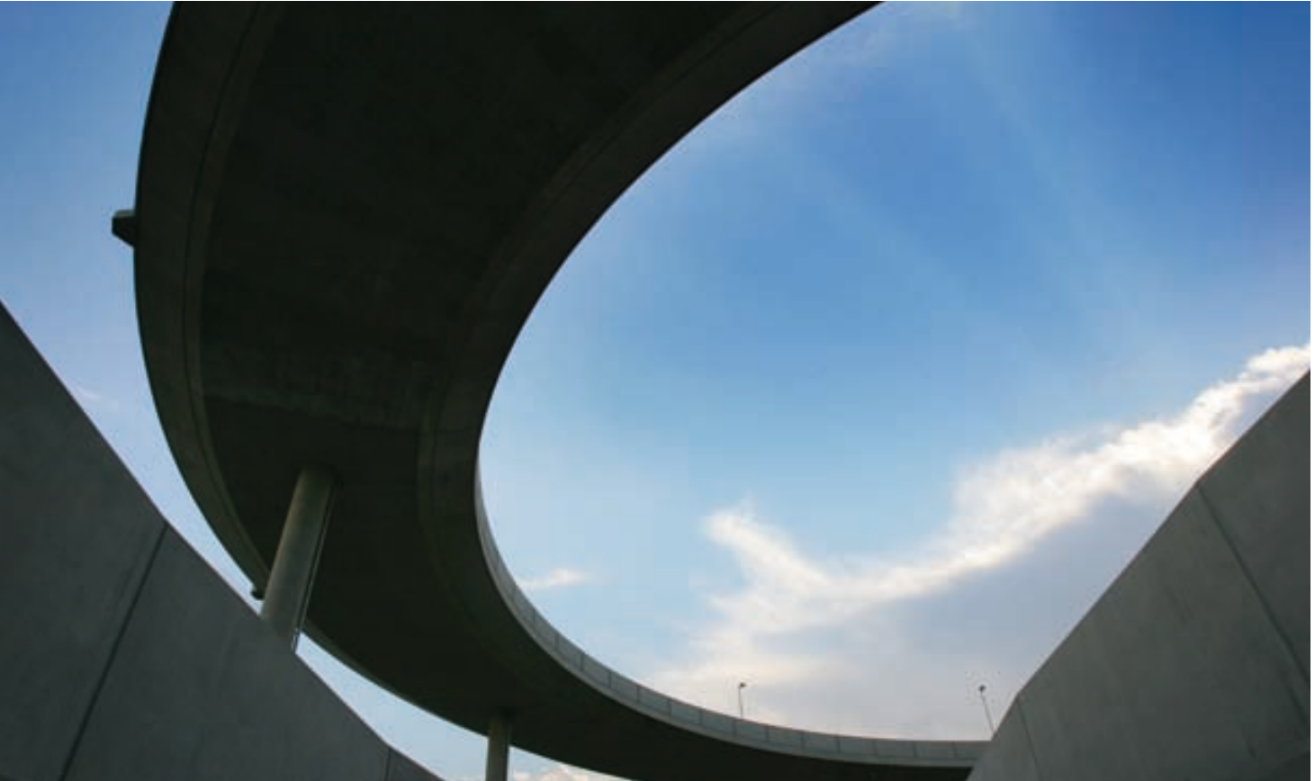
Access ramp to Heathrow Airport (London, United Kingdom)
