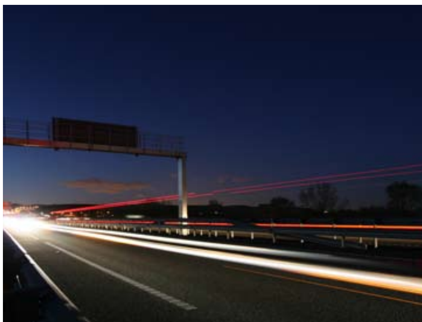
Radial R-4 Toll Road (Madrid, Spain)
