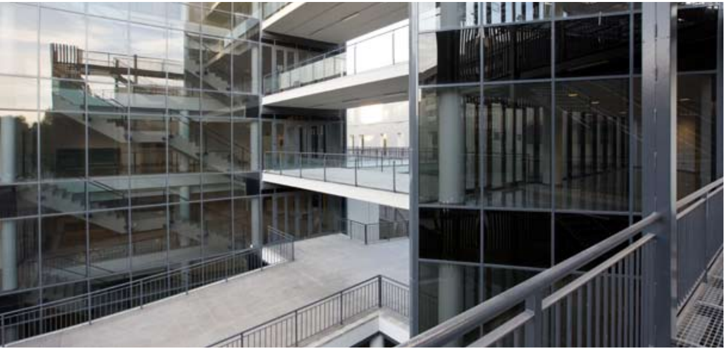
Faculties of Law and Work Sciences at the University of Seville, Spain
