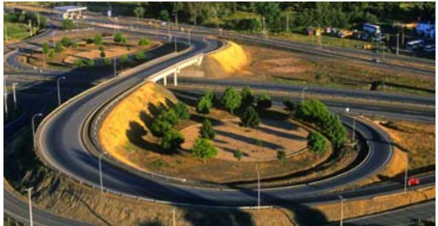
Aerial view of one of Cintra's Chilean toll roads
