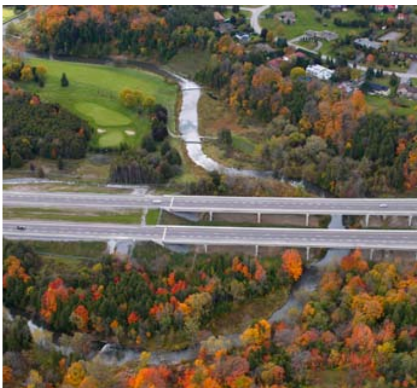
407 Express Toll Route (Toronto, Canada)
