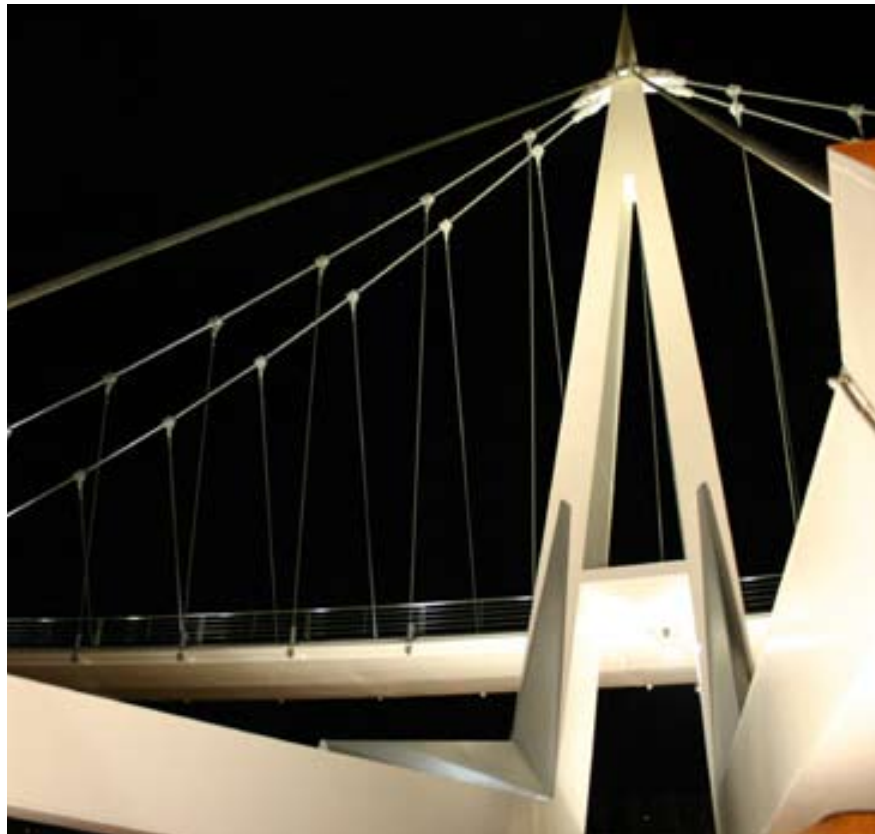
Footbridge in Delicias (Zaragoza, Spain)
