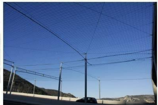
Detail of the protection structure of the bat passageway
