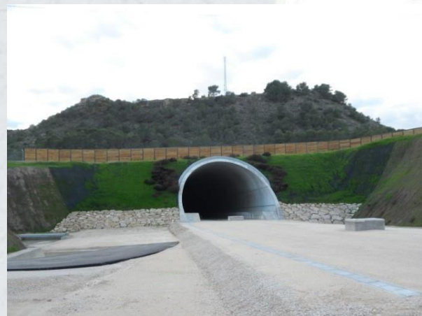
Tunnel outlet stabilisation work
