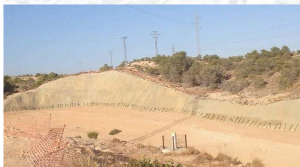
Appearance of the slopes to be restored
