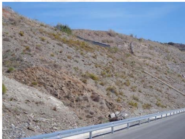
Dismantling in the process of recovery
