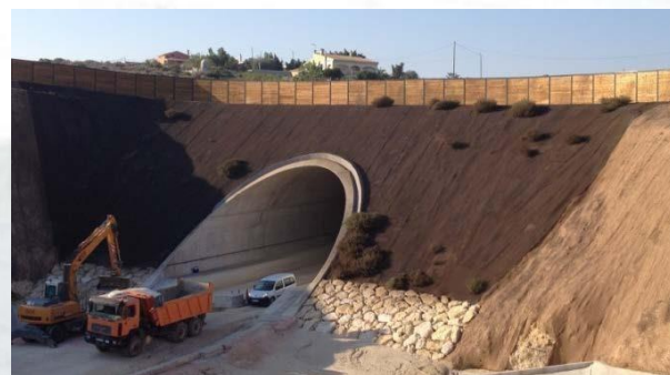
Tunnel embankment with riprap footing and hydroseeding substrate
