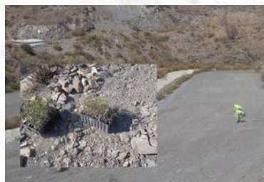
Planting work (detail of cuttings)
